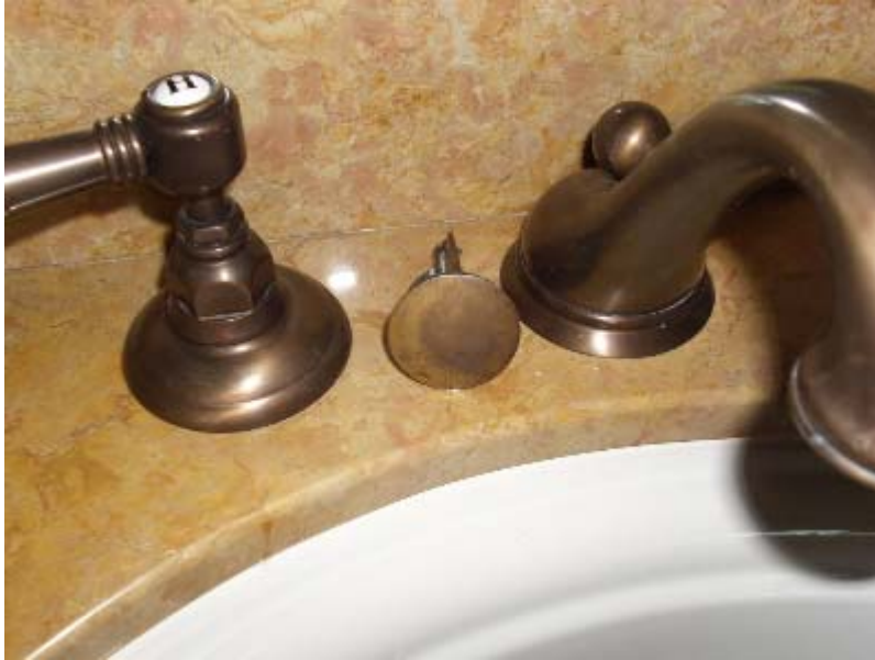
Drain stop needs repair
